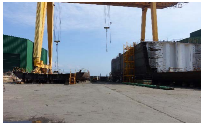
Hull 33 and 34 on slipway (hull 33 on the left, hull 34 on the right).
